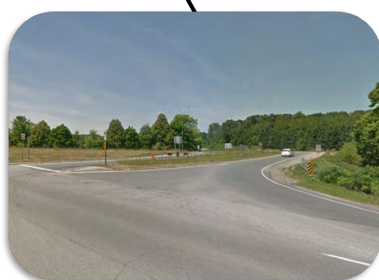
402 Ramp at Glendon Drive
