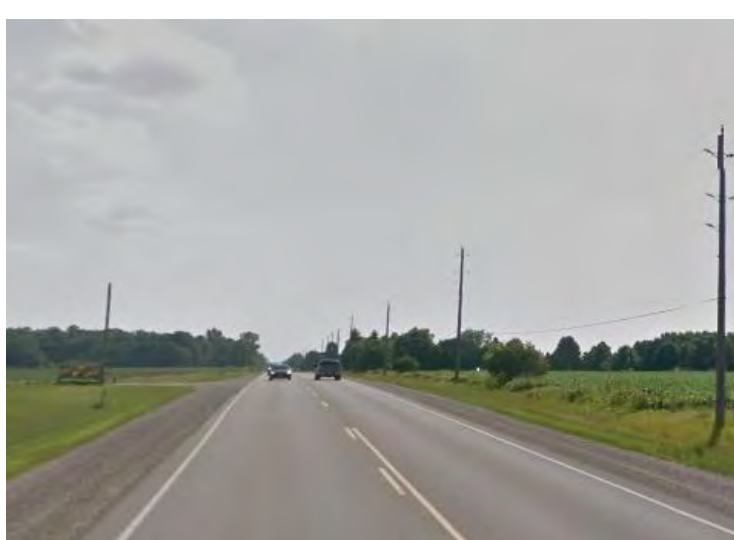
Road section at Vanneck Road
