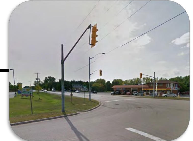
Komoka Road at Glendon Drive
