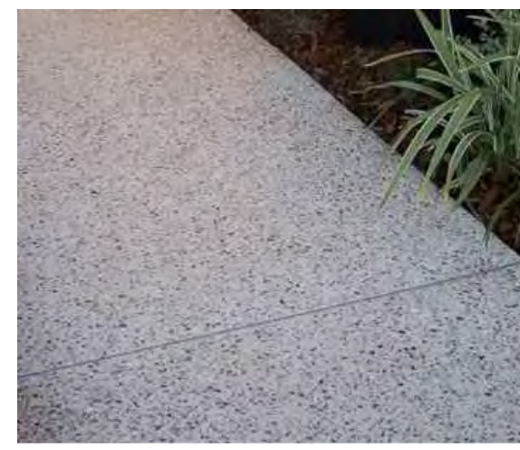
EXPOSED AGGREGATE PAVING
