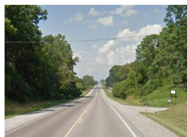
Road section at Komoka Creek
