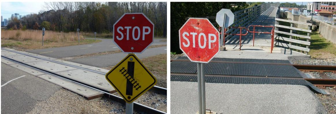
Track Crossing Material Alternatives to Asphalt (Left: Concrete) (Right: Rubberized Matting)
