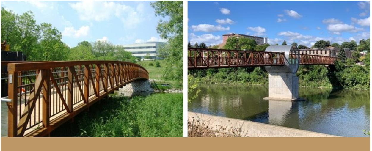
PHOTOS OF PONY TRUSS AND H-SECTION BRIDGES
